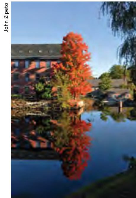
Ballardvale Dam, Andover
